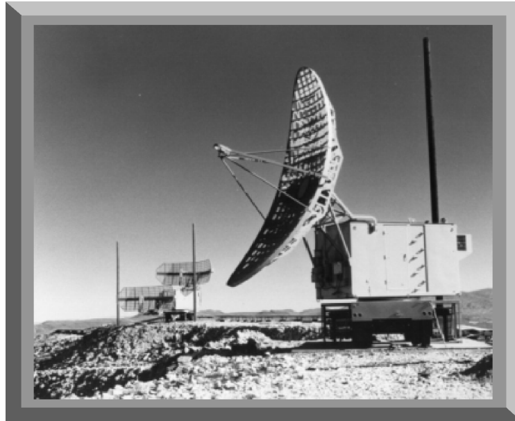
Figure 6-3. Height-Finder Parabolic Antenna
